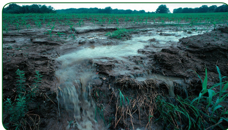
Poor soil aggregation tends to form surface crusts and compacted surface soil. This can reduce water infiltration and storage and lead to excessive runoff and erosion. Source: indianapublicmedia.org
